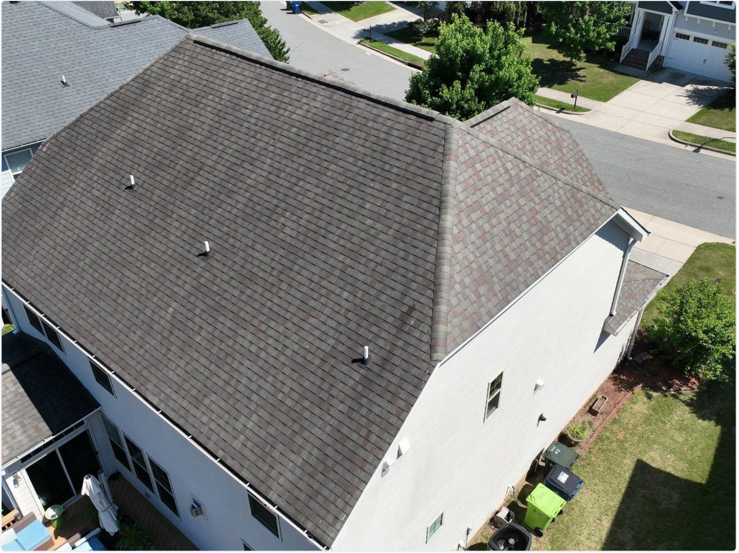
Fig. 2 — Oblique across the front planes; uniform shingle field and continuous gutter line.
