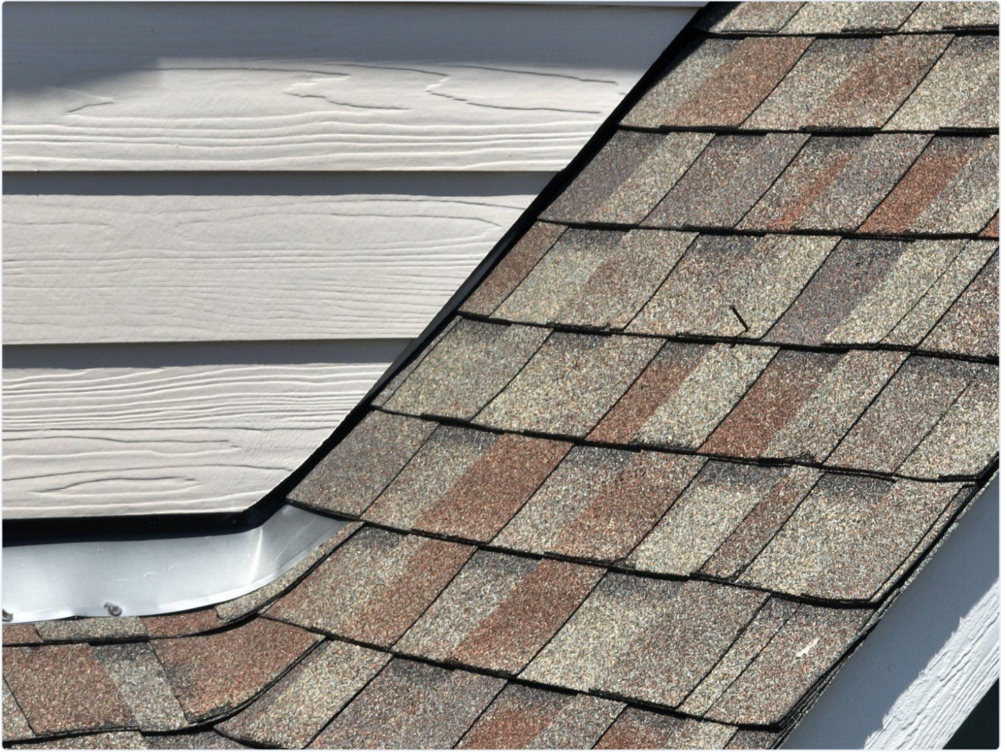
Fig. 4 — Shingle field at close range; courses uniform, no lifted or missing tabs observed.
