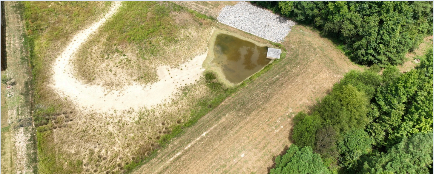
Fig. 7 — Outlet structure and channel at closer altitude; grate clear, surrounding vegetation established.
