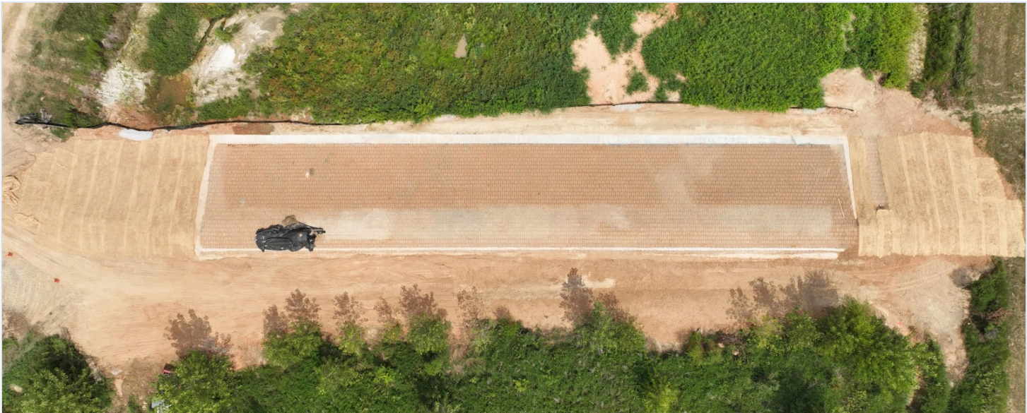
Fig. 8 — Maintained path; graded running surface and defined shoulders.
