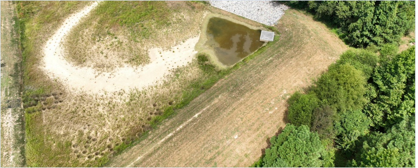
Fig. 6 — Stormwater control measure. Forebay with sediment accumulation, permanent pool, outlet structure and rip-rap emergency spillway.
